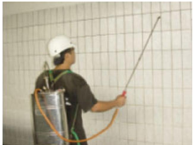
**Fig. 493: Disinfection of walls by using portable spray equipment. For operator's protection gloves and facemask are recommended.**
