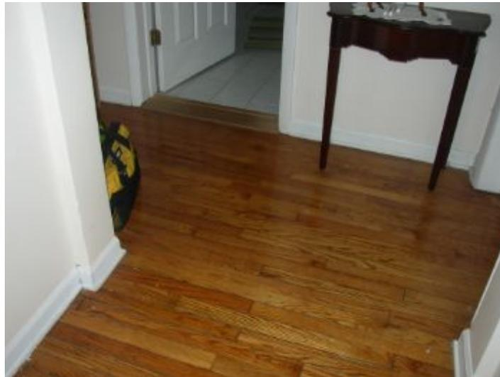
The 1st floor is sagging in hallway by the bathroom. Master bedroom doors have large gaps on one side. Recommend further evaluation from a contractor or structural engineer.
