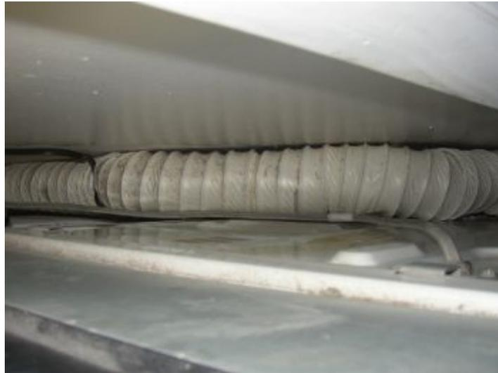
Dryer vent hose should be solid metal type. Plastic could burn and foil corrugated type clog easily.
