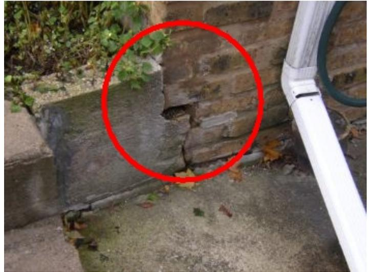
Missing/Deteriorated mortar observed, suggest tuckpointing as necessary.
