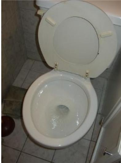
The toilet bowl is loose at floor 2nd floor. The wax ring inside the unit must have a snug, secure fit in order to keep from leaking. Properly resealing and re-securing this unit is suggested to prevent water leakage and damage to the sub-floor area.
