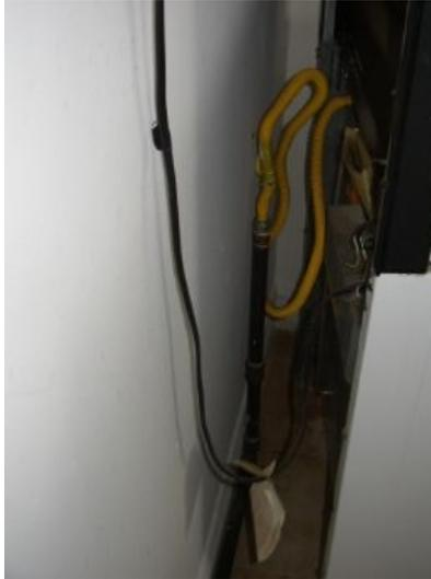
Gas valve missing at gas service pipe (2nd floor). Manual gas shut off valve required at each appliance.
