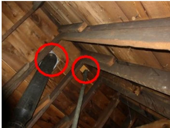
Light shows through the plumbing vents which may indicate a leak. Repair flashing
