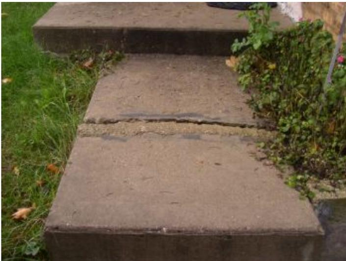
Cracks and heaved/settled areas observed by front door. Eventual replacement is recommended
