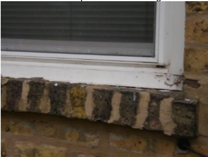
Some brick windows sills are pitched toward the house allowing water to pool and possible water intrusion into the walls
