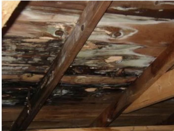
Evidence of water penetration observed and roof sheathing is rotted.
