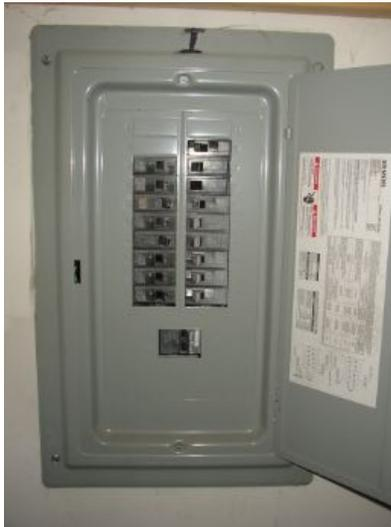
There are three 20 amp circuit breakers with 14 gauge wires. Either install a 15 amp breaker or replace ALL 14 gauge wire with 12 gauge wire.1st floor panel
