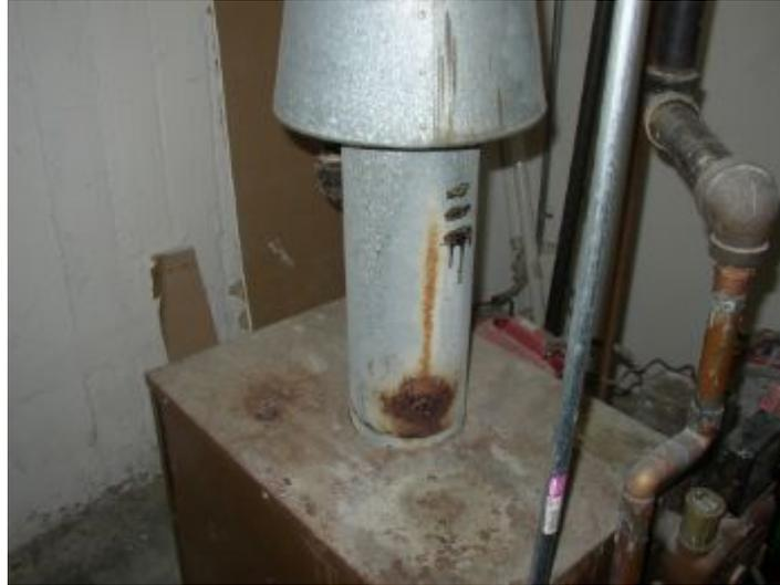
Holes/ rust observed in flue vent pipe for boiler, which is a serious safety concern. Replace all flue piping, installed w/ screws in each section.
