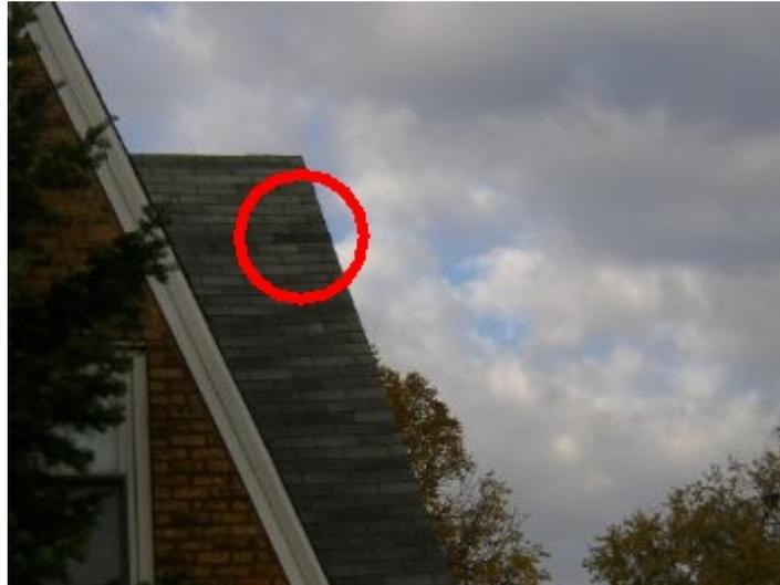
Some shingles have damage or have blown off. The roof is past its expected life. Recommend replacement
