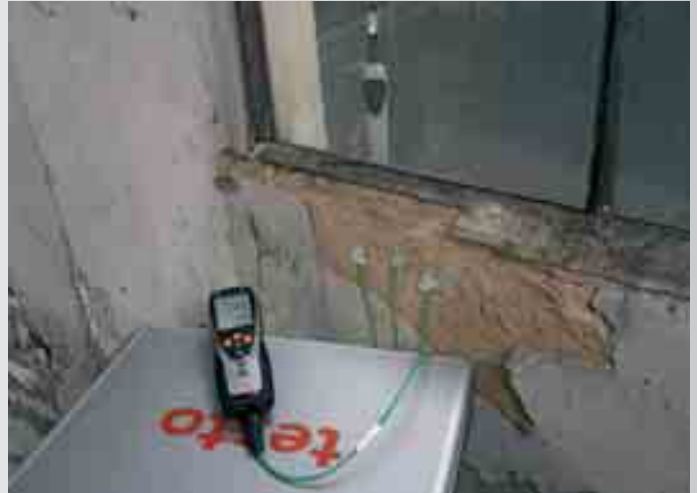
Measures the U-value in a wall in need of renovation using U-value and wireless temperature/humidity probe (alternatively conventional temperature probe also)
