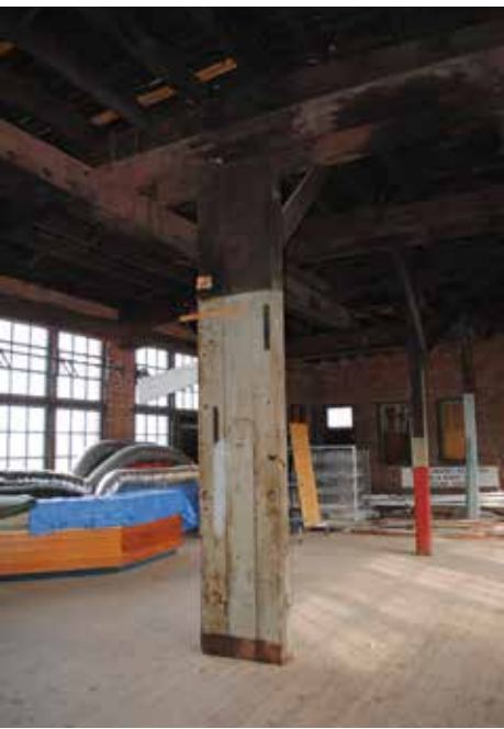
Car Shop Before
