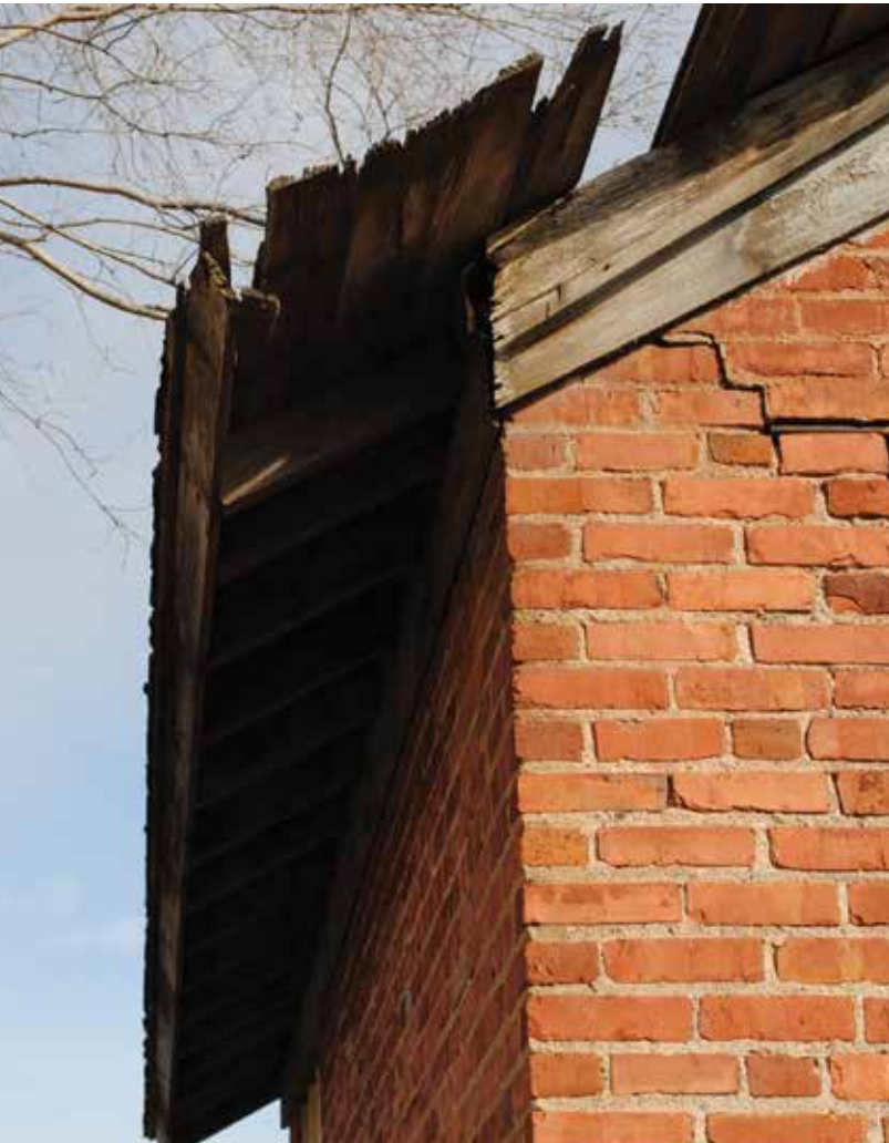
Water Closet Roof Before
