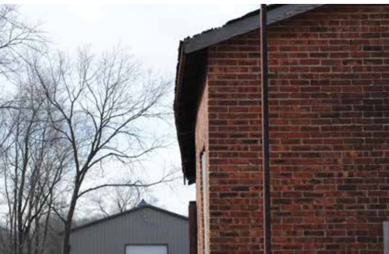
Sandhouse Wall Before
