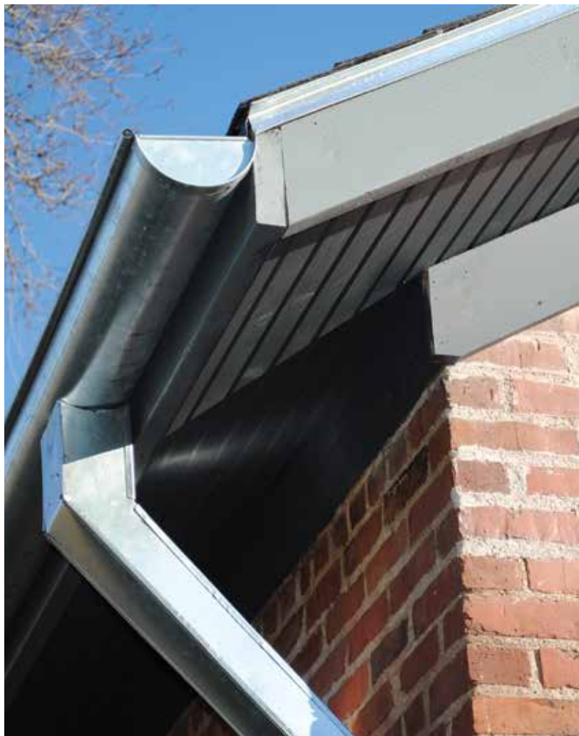
Water Closet Roof After
