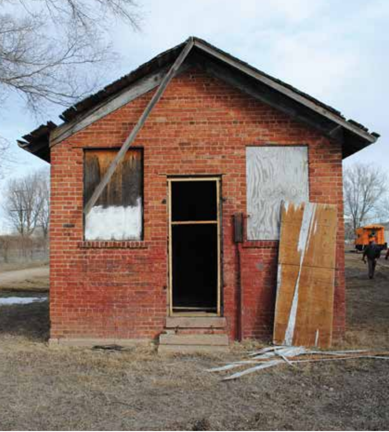
Water Closet Before
