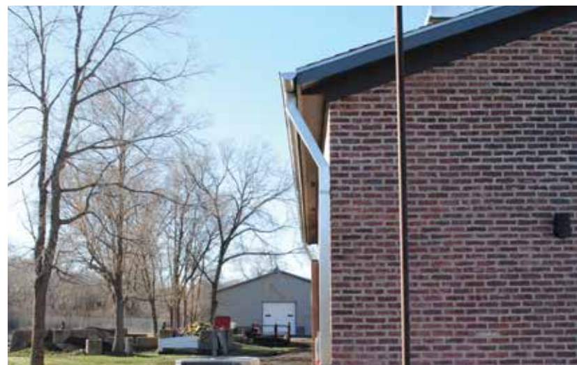
Sandhouse Wall After
